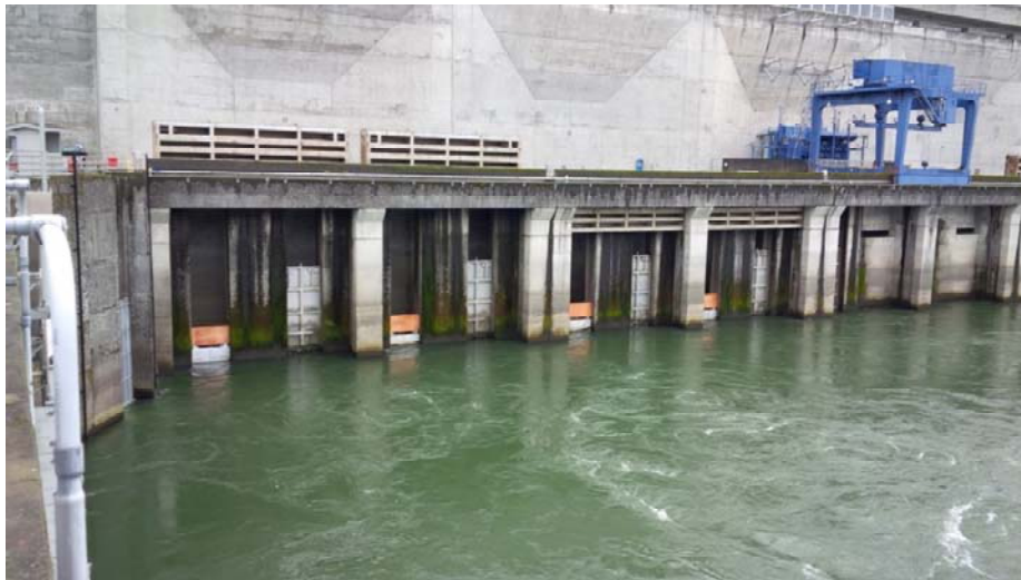
Figure 6. Bonneville Dam powerhouse 2 tailrace view of the FOGs with additional wooden panels installed on February 29, 2016 to prevent sea lions from jumping into the fishway.
