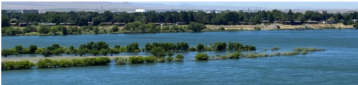
Figure 1. Flooding at the northern end of Island 20 on June 28, 2022.
