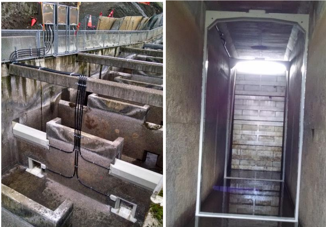
Figure 10 New PIT-detection Arrays in the Lower and Upper Lower Granite Dam Fishway, 2016
