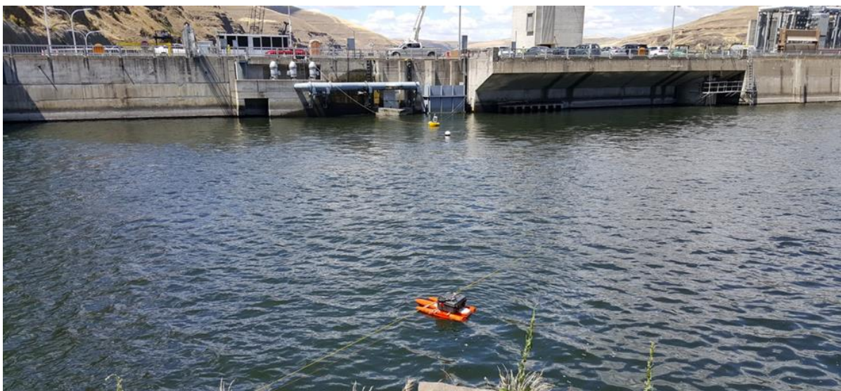
Figure 16 Photograph of Temperature Control Structure Turned Off
