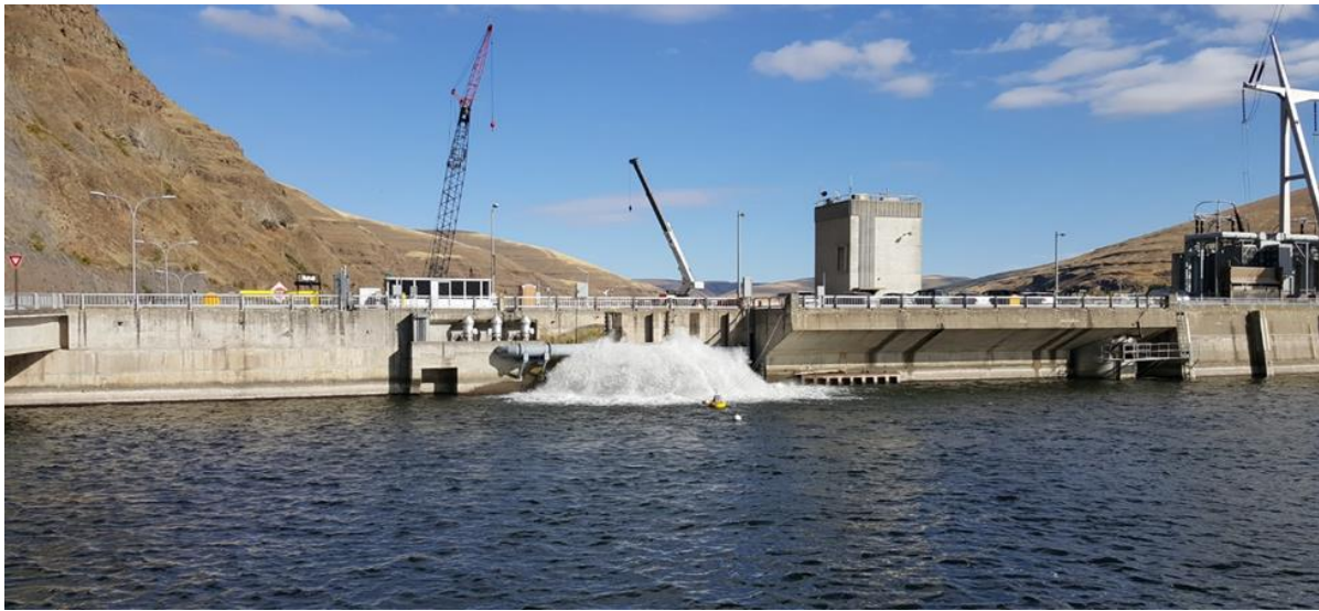
Figure 15 Photograph of Temperature Control Structure Turned On
