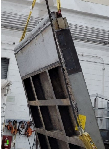
Figure 3: Picture of the steel plating installed on the downstream face of the newly modified SE-1 weir. The flat surface will provide an attachment point for lamprey before entering the SFL.
