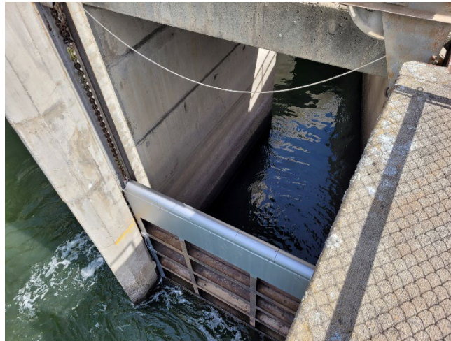
Figure 4. newly modified SE-1 weir installed.
