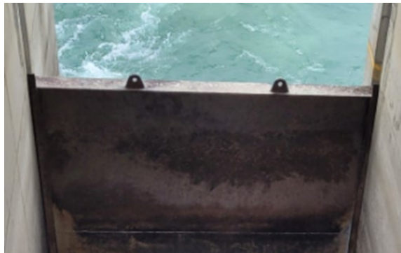
Figure 1: The currently deployed SE-1 top. The flat surface makes it difficult for lamprey to enter the system.
