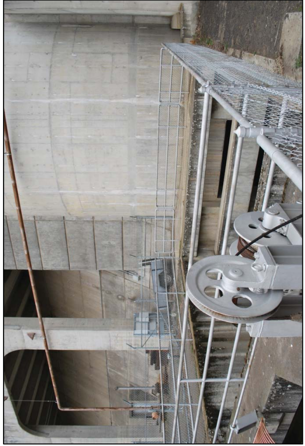
Photograph 11. Location at ground level.
