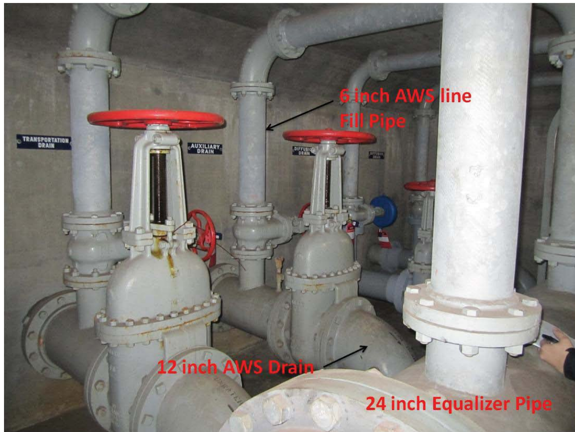
Figure 6. AWS Drain and Equalizer Header Pipe Connection
