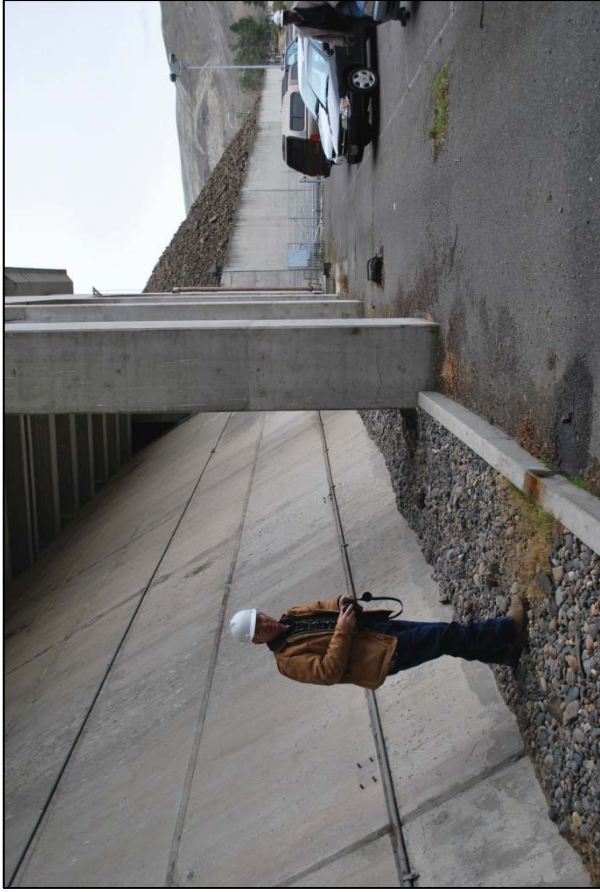
Photograph 12. Potential alignment into pipes or Low Level Intake.
