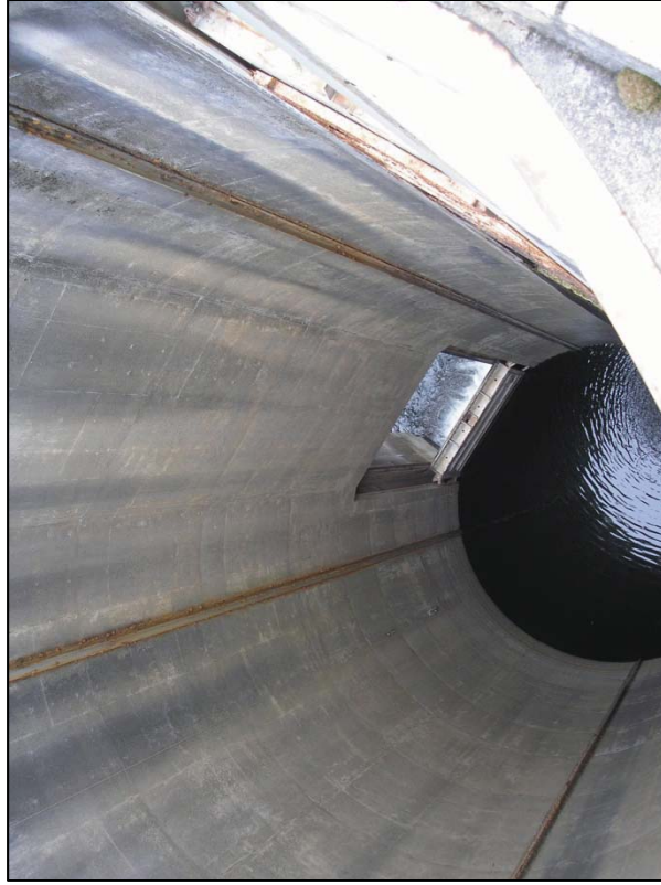
Photograph 5. Interior view of the dam structure.
