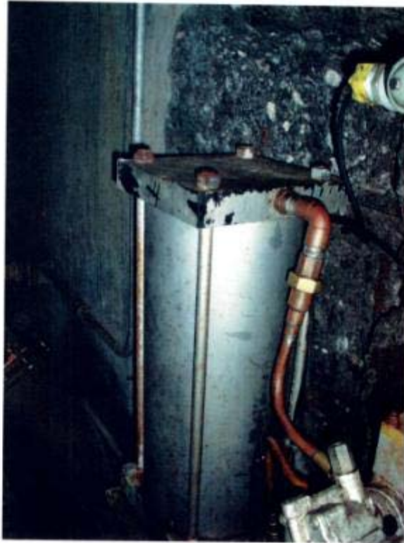
Photo 1: Grey Actuators With Concrete Chipped Away - All Alternatives. Offset = 0.6 inches
