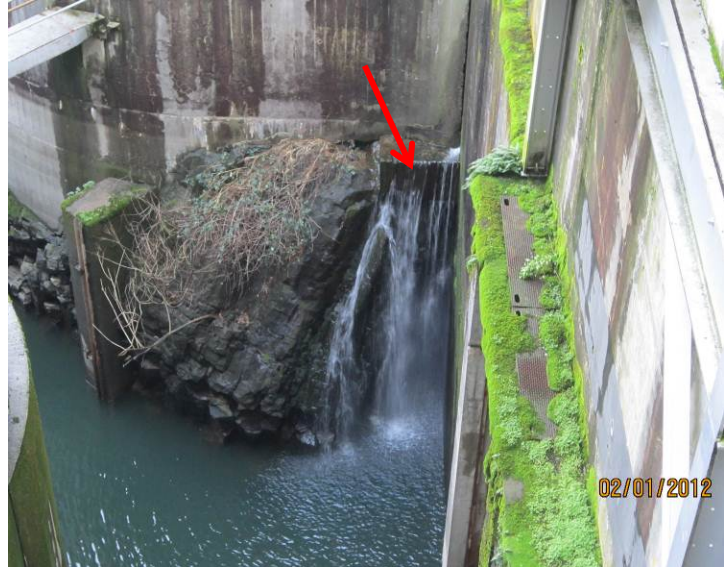
Figure B2.4.11 Channel between Fish Lock and Collection Channel
