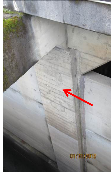
Figure B2.4.5 New Concrete Below Joint
