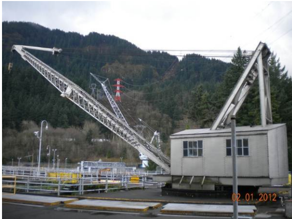
Figure B2.4.26 Crane at South AWS Intake
