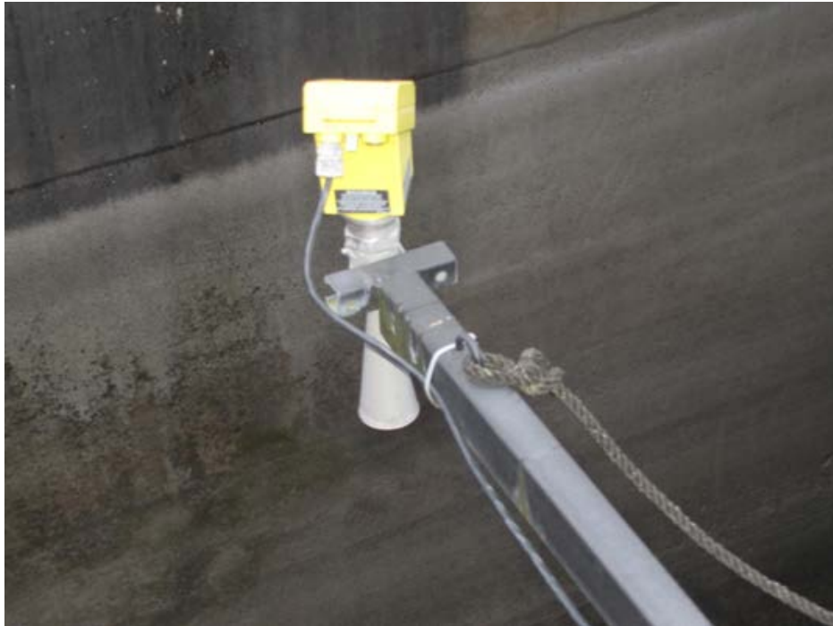
Figure B1.6.1 Radar Level Transmitter/Receiver
