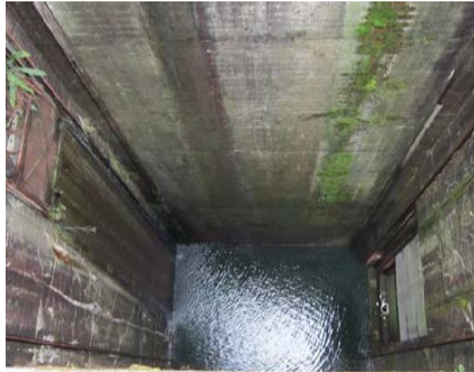
Figure B2.4.7 Fish Lock Chamber
