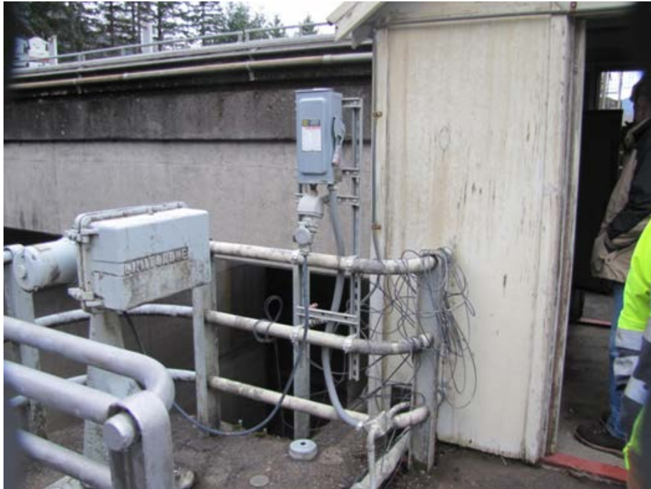
Figure B1.6.6 Limitorque Operator with Disconnect Switch
