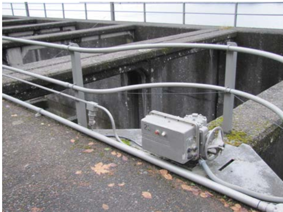
Figure B1.6.7 Limitorque Operator without Disconnect Switch
