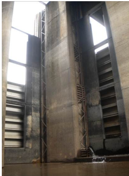
Figure B3.4.1 Fixed Weirs (SO-SG-2 and SO-SG-7)
