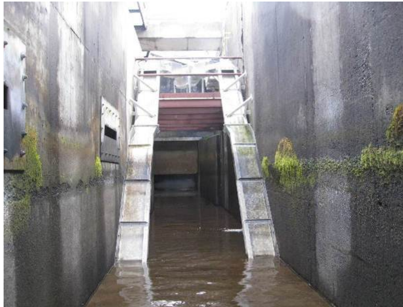
Figure B2.4.23 Lamprey Bypass in the Makeup Water Supply Channel
