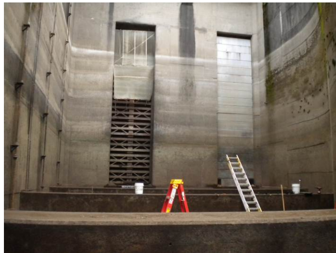
Figure B3.4.3 Channel to Fish lock with Fish Lock Bulkheads in Background
