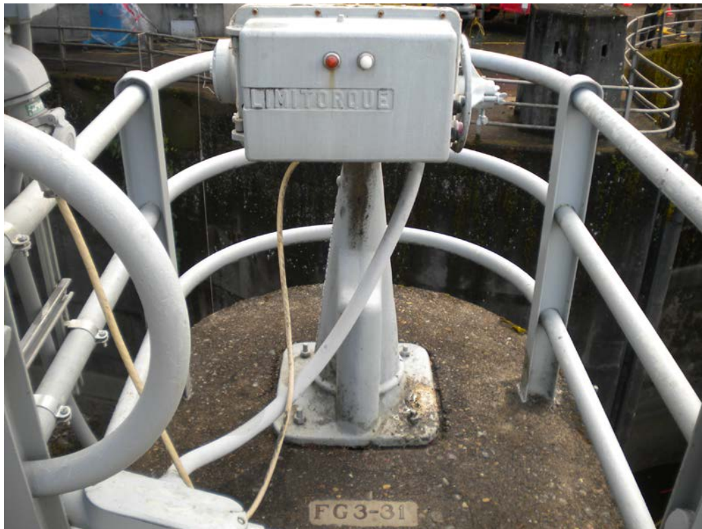
Figure B3.4.10 Limatorque Gate Actuator for FG3-31
