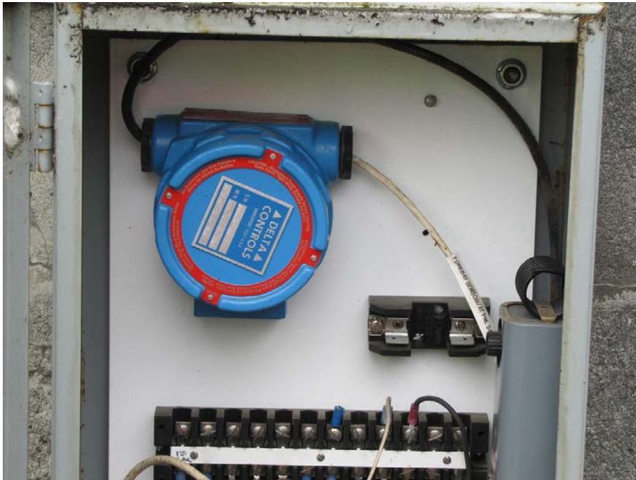
Figure B1.6.3 Level Transducer Converts Pressure Signal to 4-20mA for Input to PLC
