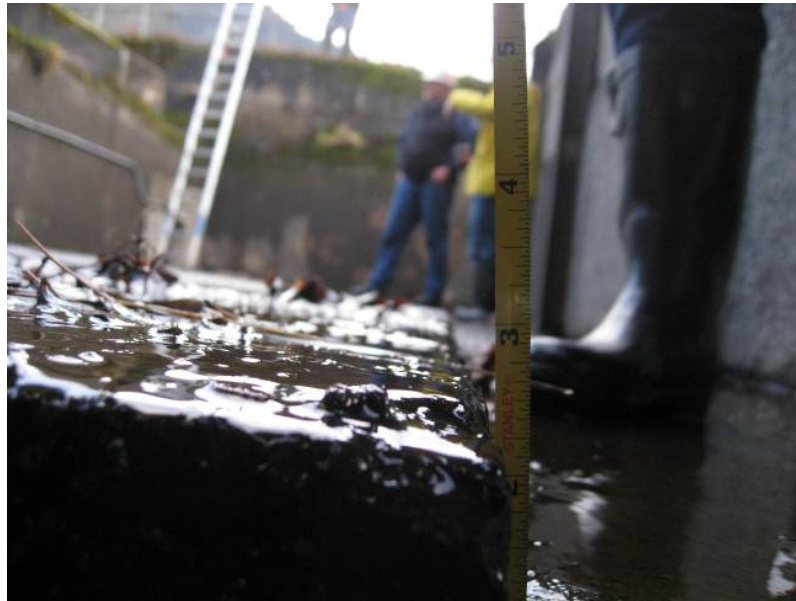
Figure B2.4.16 Raised Replacement Concrete Slab
