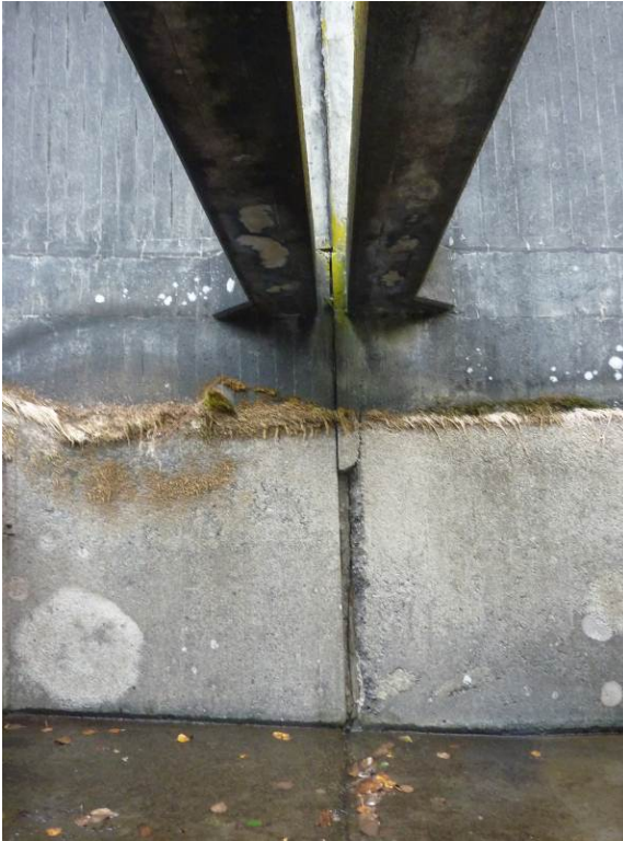
Figure B3.4.4 Expansion Joint between Weirs 37 and 36.
