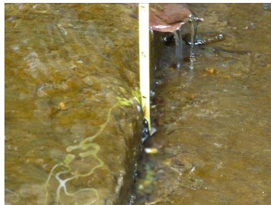
Figure B2.4.15 Raised Replacement Concrete Slab
