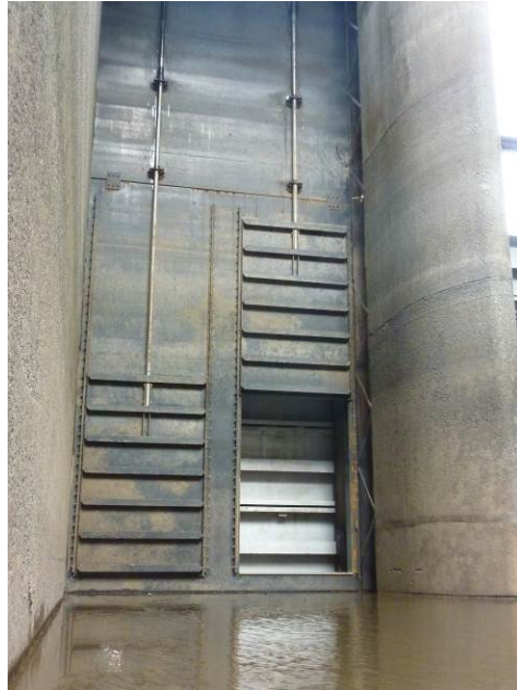
Figure B3.4.2 Sluzice Gates (SW-SG-4N and 4S)
