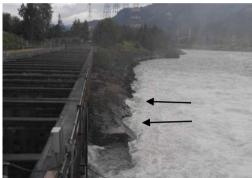
The ROV survey on 17 June showed erosion but no undercutting of the fish ladder at this time (details are available in **16BON32 attachment 1**).
