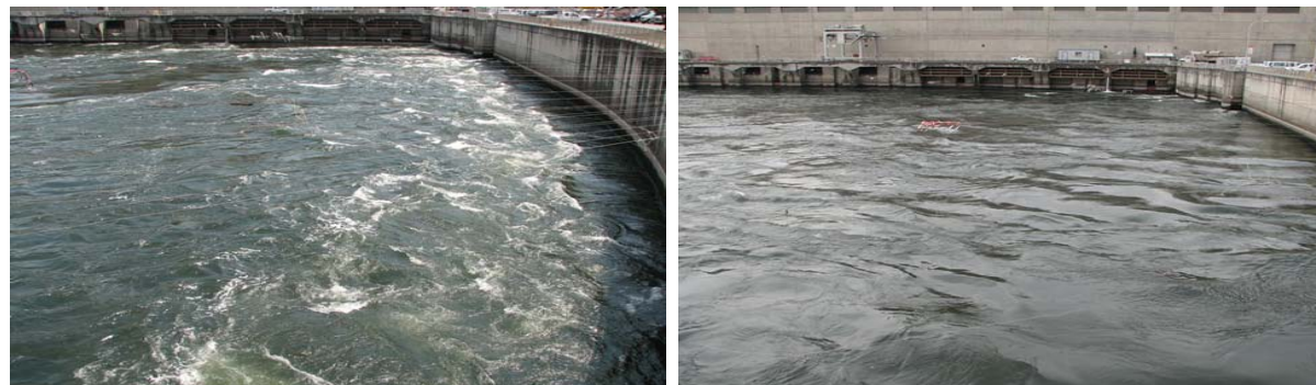
Figure 1. Tailrace conditions at Lower Granite Dam July 2013 with upstream flow during FPP operation (left) and downstream flow during Unit 1 operation (right). Photo courtesy of Darren Ogden 2013.
