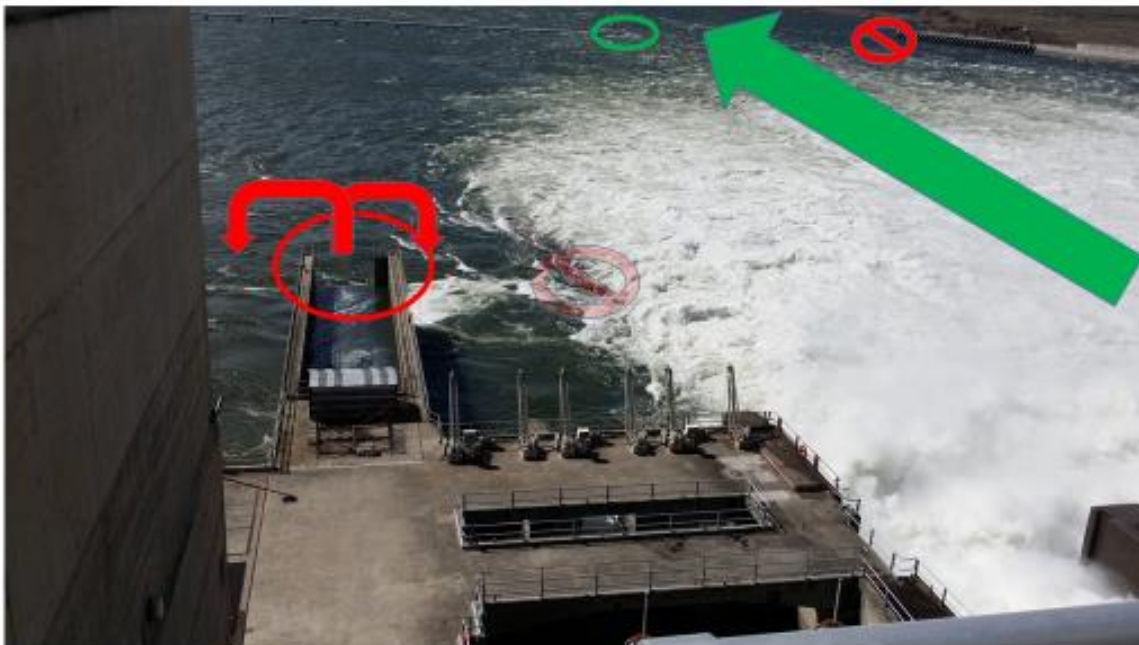
Figure 1. Photograph illustrating McNary Dam tailrace during spill operations and different pathways expected during different fish passage operations. The green circle (top center) is the primary and secondary outfall for bypassed fish, and the green arrow (top right corner) represent the primary top spill weir jet created for use by spilled fish. These green references show passage routes expected in 2021 regulatory documents. The spill pattern simulations at ERDC, in part, emphasized a design that minimized encounters in the red crossed-out circle at the top right. In addition, the spill pattern simulations at ERDC emphasized a design that minimized the encounters with the strong transition areas and eddying (faded red crossed out circle in the center), including the location of past debris. Both these areas were strongly emphasized as the least desired areas for emigrating fish. The red circle with emphasized arrows (middle left) represents the point every emergency bypassed fish is entering the tailrace with emphasis on the flow vectors that each can face.
